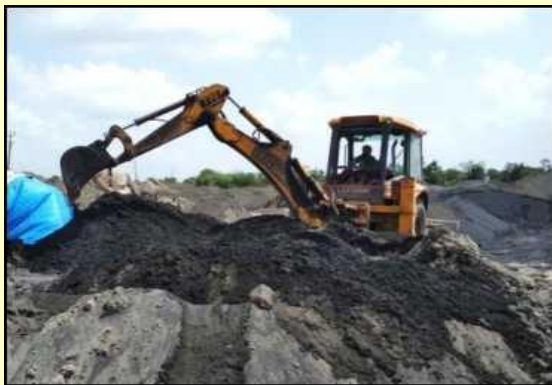
Wet mixing of copper slag and fly ash mixture
