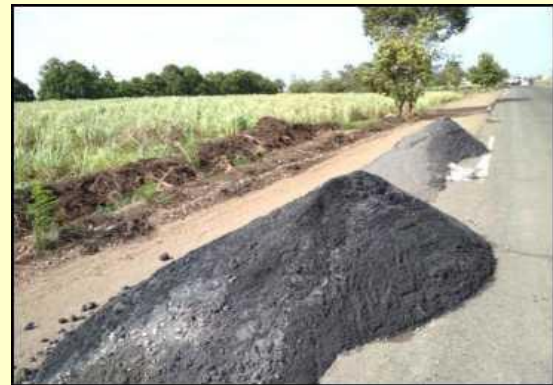
Stacking of the mix on subgrade
