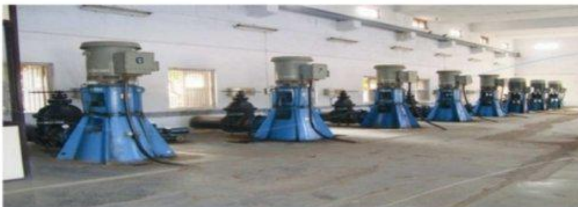
V.T. PUMP SETS INSTALLED AT SMC WATER DISTRIBUTION STATION
